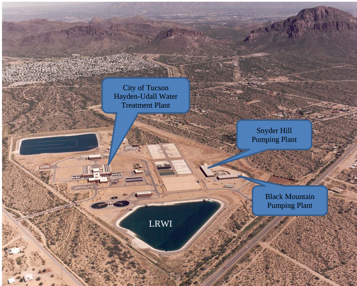
Figure I-3– Snyder Hill and Black Mountain Pumping Plants
